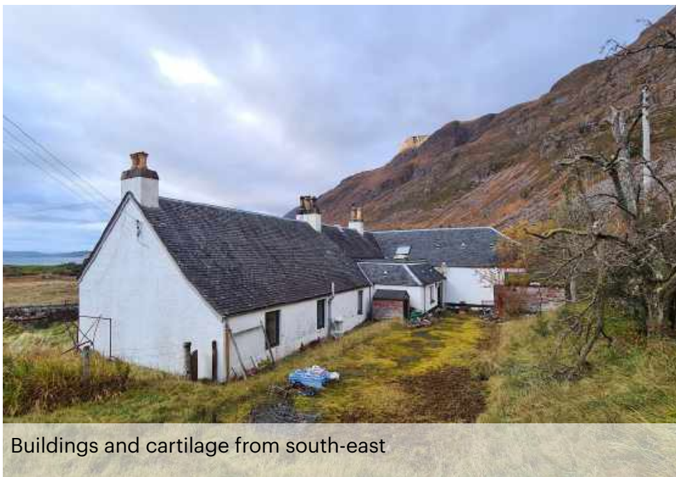
Land and building from north
