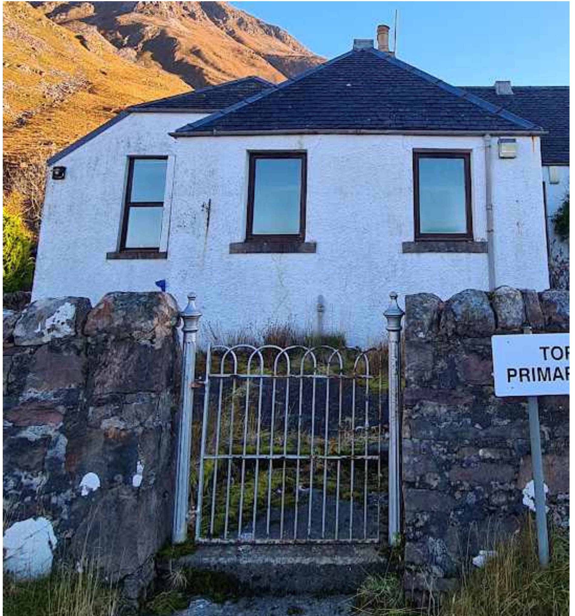
Externals: gate and stone wall condition
